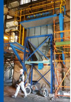
New extraction units will eliminate sugar dust in the packing and sugar bin areas.
